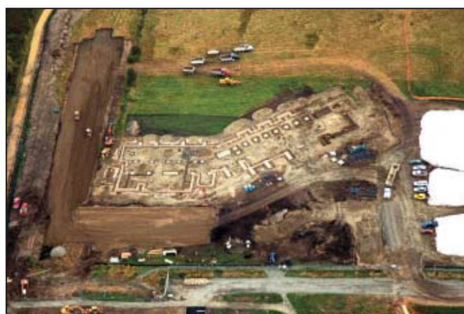
The building's footprint begins to take shape.
