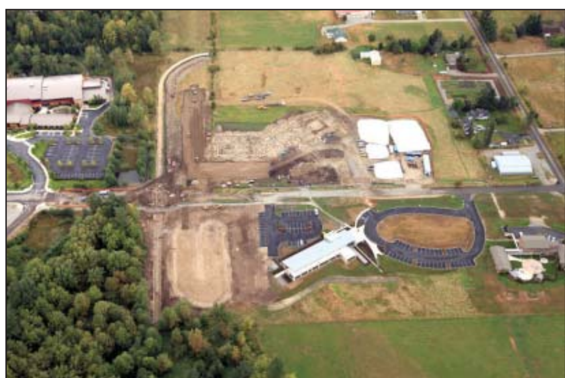
Aerial View of the site, with Health & Wellness Center at left and Behavioral Health in the foreground.
